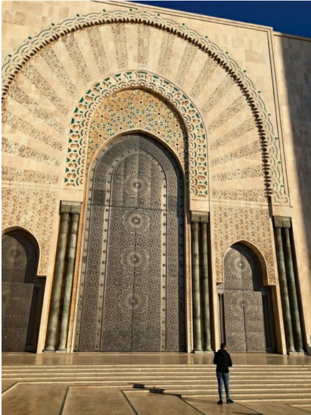
Zellige mosaic tiles adorn the exterior of the Hassan II Mosque designed by a French architect and opened in 1993.
