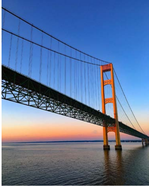
Passing under Mackinac Bridge at dawn aboard Victory I during a Great Lakes cruise. Photo by Katherine Rodeghier
